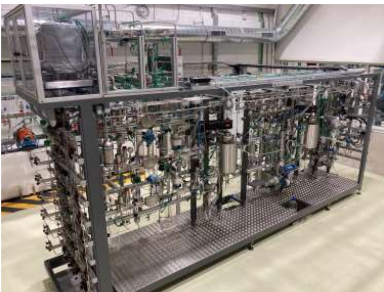
Vinci's pilot plant for Hydrothermal Liquefaction HTL of biofeed
